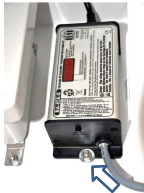
Figure 4. Press reset button on side of ballast while pump is running.
