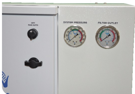
Switch to Manual 'MAN' Position
