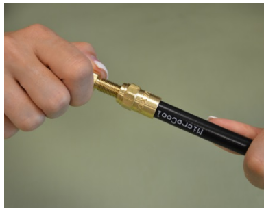
Figure 8: Screw Stem into Ferrule
